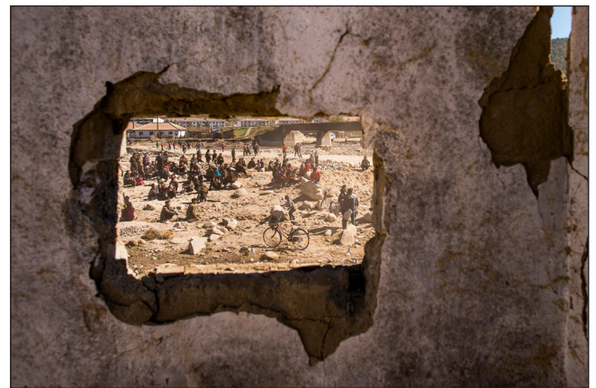
Yonsa flood destruction, 2016.
