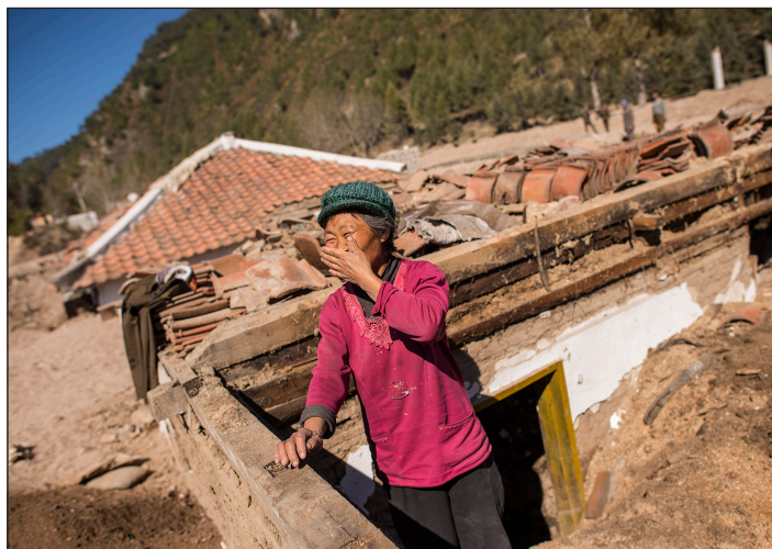
Mud filled the houses as the river washed out the valley.
