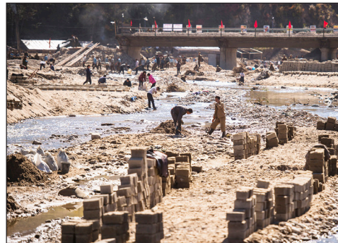
Rebuilding Yonsa after a storm in 2016.
